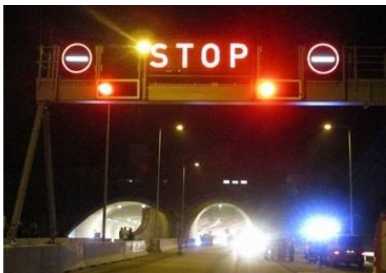
Figure 6. Lane control signs and variable message signs at tunnel portal
